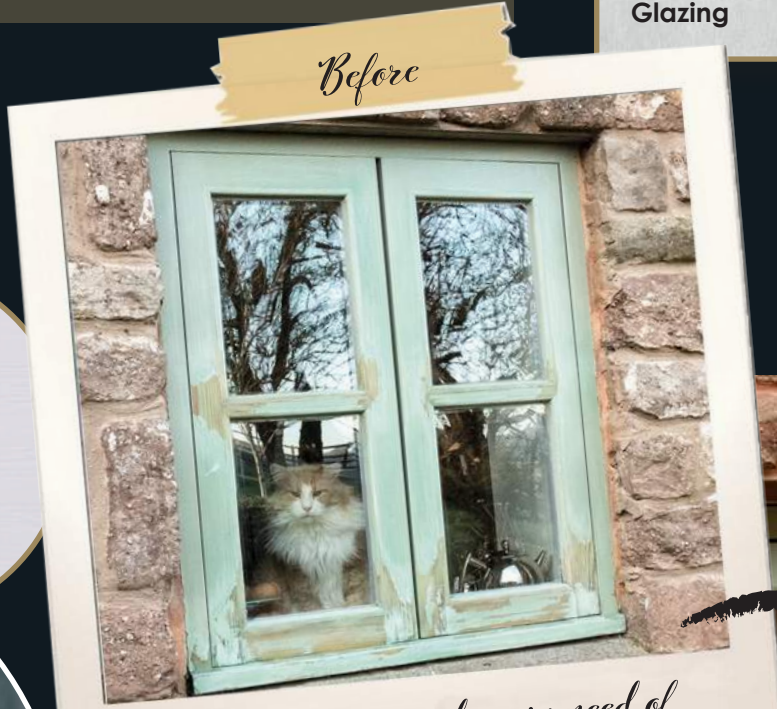
Rotten timber windows in need of some serious repair & maintenance
